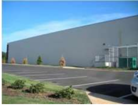
Figure 64 A – Not permissible
