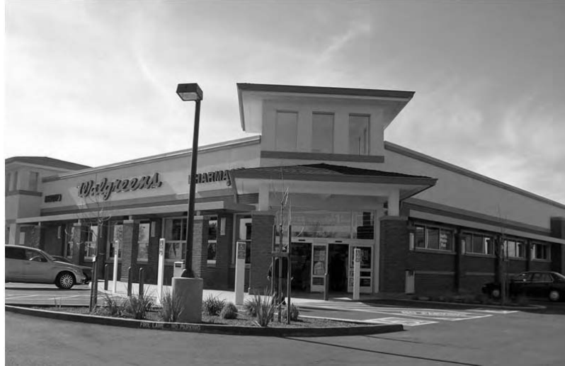
Figure 69 Example of appropriate treatment of a corner building
