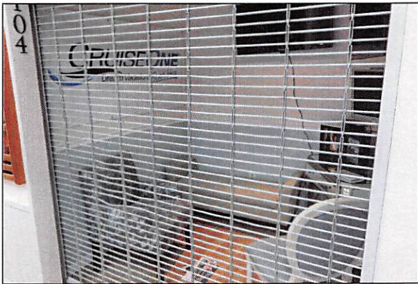
Former elevator shaft; rental nook to Travel Agency
