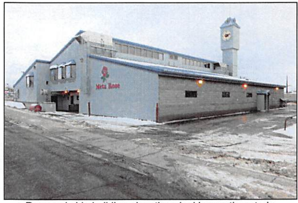
Rear and side building elevations looking northeasterly
