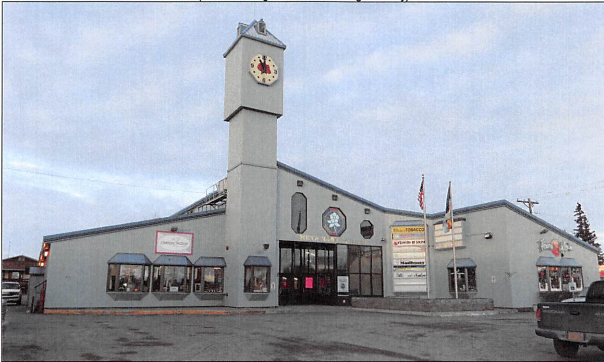
(front building elevations looking westerly)
