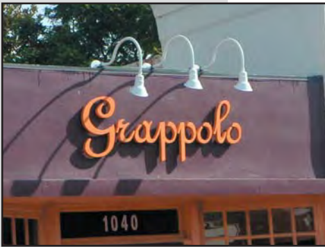
GOOSE-NECK STYLE LIGHTING IS AN ATTRACTIVE WAY TO LIGHT SIGNAGE.
