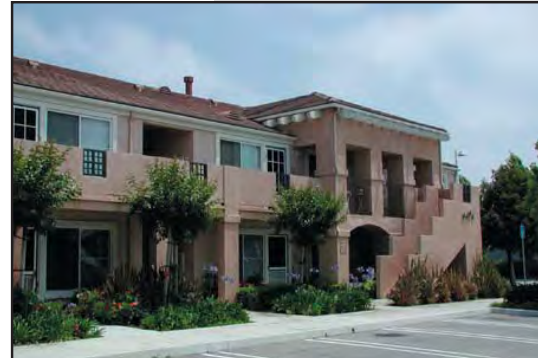
SIMPLE, CLEAN, BOLD PROJECTIONS OF STAIRWAYS SHALL BE USED TO COMPLEMENT THE ARCHITECTURAL MASSING AND FORM OF MULTI-FAMILY STRUCTURES.
