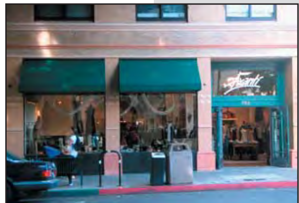
AWNINGS SHALL BE PLACED WITHIN VERTICAL ELEMENTS WHEN THE FACADE OF THE BUILDING IS DIVIDED INTO DISTINCT STRUCTURAL BAYS.
