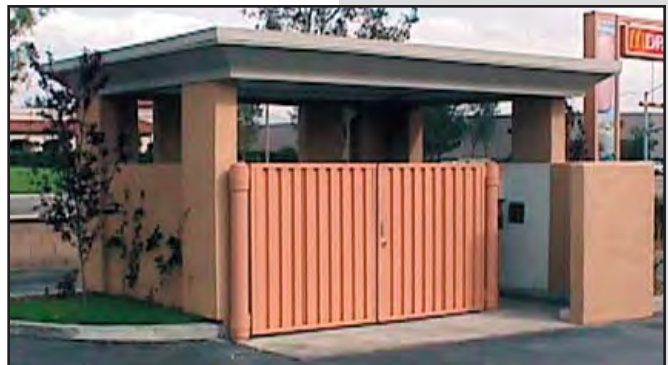
A PEDESTRIAN ENTRANCE TO THE TRASH ENCLOSURE SHALL BE PROVIDED SO THAT THE LARGE ACCESS GATES DO NOT HAVE TO BE OPENED AS OFTEN.
