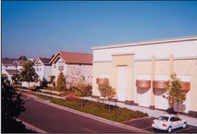
LANDSCAPE BUFFERS AND BUILDING ARTICULATION HELP TO EASE THE TRANSITION BETWEEN INDUSTRIAL AND RESIDENTIAL BUILDINGS.
