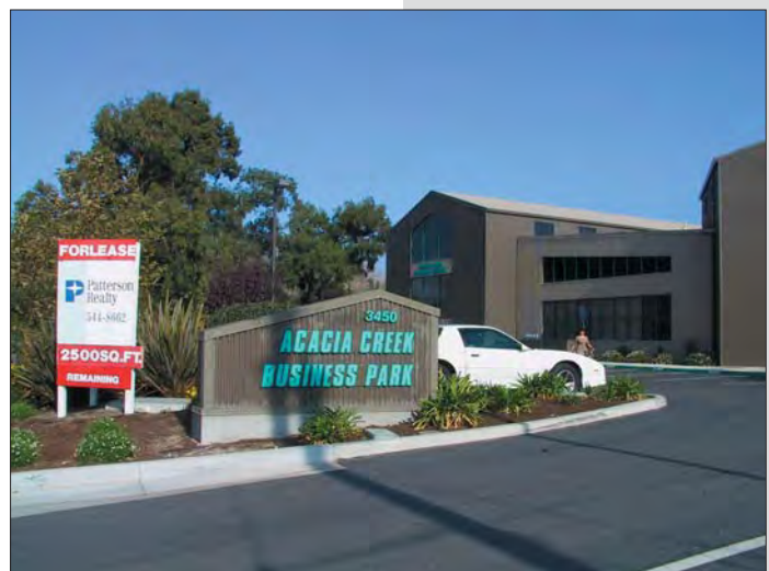
MONUMENT SIGNS THAT INCORPORATE SIMILAR MATERIALS AND COLORS AS THE CORRESPONDING BUILDING ARE ENCOURAGED.
