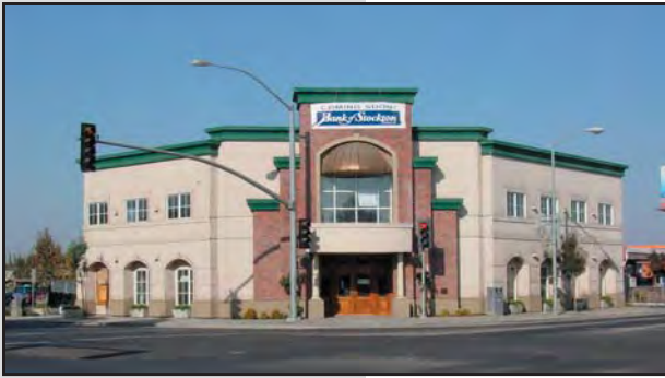
SPECIAL ATTENTION SHALL BE GIVEN TO BUILDING ORIENTATION AND ARTICULATION ON CORNER SITES.
