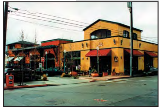
DETAILS SUCH AS WALL SURFACES CONSTRUCTED WITH PATTERNS, CHANGES IN MATERIALS, BUILDING POP-OUTS, COLUMNS, OR RECESSED AREA TO CREATE SHADOW PATTERNS AND DEPTH ON THE WALL SURFACES SHALL BE USED
