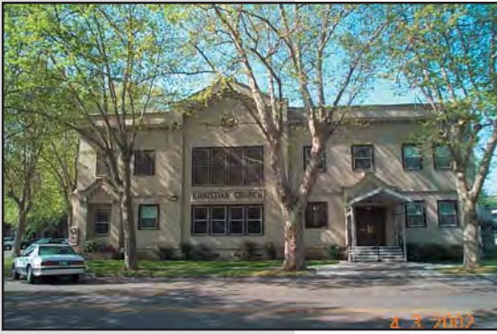
PARAPETS SHALL HAVE SUFFICIENT ARTICULATION OF DETAIL SUCH AS PRECAST TREATMENTS, CONTINUOUS BANDING OR PROJECTING CORNICES, LENTILS, CAPS, CORNER DETAILS, OR VARIETY IN PITCH.
