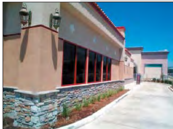
THE USE OF MATERIALS AND COLORS USED HERE HELPS DEFINE A BASE, BODY AND CAP.
