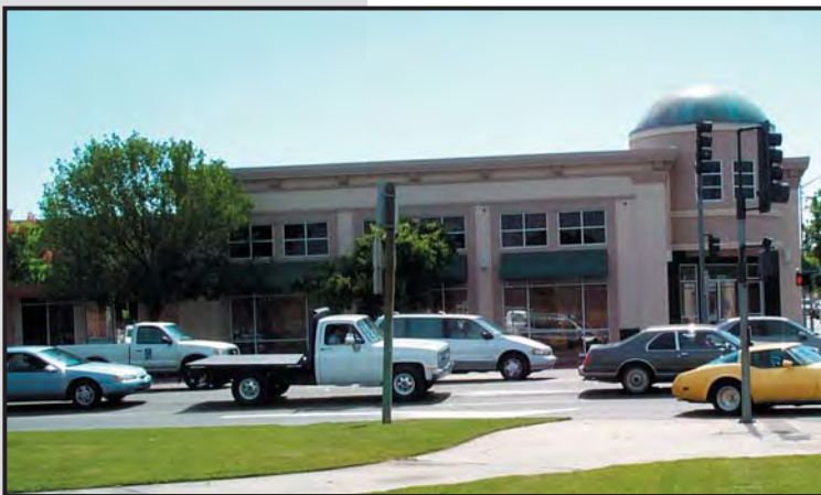
DESIGN ELEMENTS SUCH AS PARAPETS AND CORNER TOWERS SHALL BE USED TO ESTABLISH BUILDING IDENTITY AND CREATE A SENSE OF PLACE.
