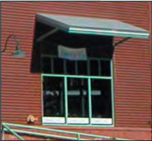
METAL CORRUGATED SIDING, METAL OVERHANGS, AND GOOSE-NECK LIGHTING MAKE THIS AN ATTRACTIVE INDUSTRIAL BUILDING
