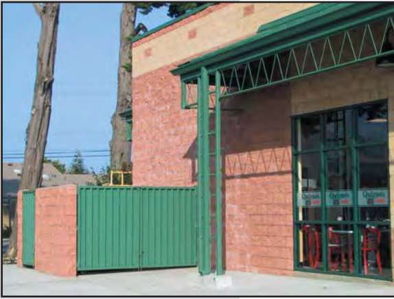
SIMILAR OF THE SAME BUILDING MATERIALS SHALL BE USED ON THE ENCLOSURE AS THE BUILDINGS
