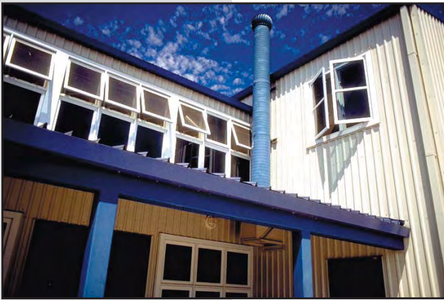
VARIATION IN WALL PLANES AND ROOF FORMS GIVE THIS BUILDING AN ATTRACTIVE FACADE.
