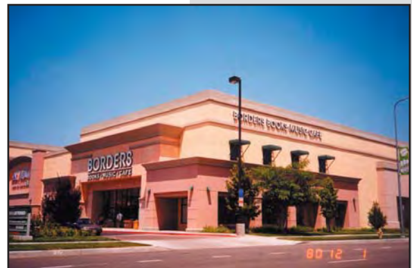
THE SCALE OF THIS LARGE BUILDING HAS BEEN REDUCED BY PROJECTING SMALLER WALL PLANES.
