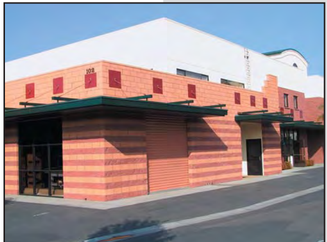
VARIATION OF BUILDING FORMS AND PLANES EMPHASIZE THE ARCHITECTURAL CHARACTER OF THE BUILDING.
