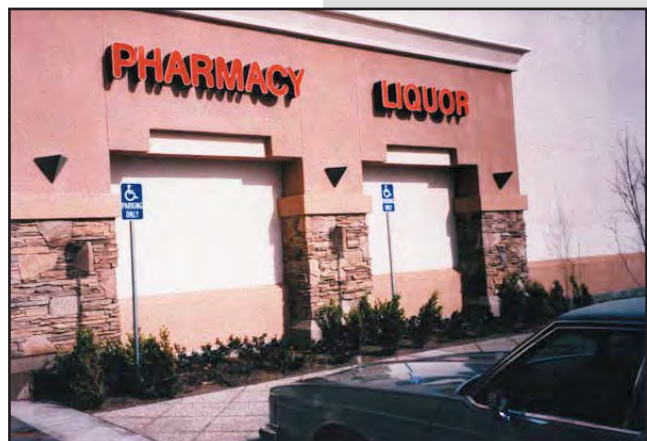
DETAILS SUCH AS COLOR VARIATION, WOOD, ROCK, OR BRICK ACCENTS SHALL WRAP AROUND THE PLANE 4' (OR UNTIL THE NEXT WALL PLANE IS REACHED).
