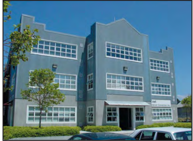
WINDOW TYPE, MATERIAL, SHAPE, AND PROPORTION SHALL COMPLEMENT THE ARCHITECTURAL STYLE OF THE BUILDING.
