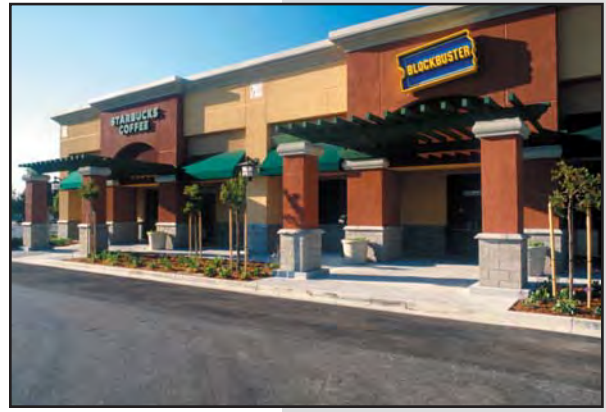
DETAILS SUCH AS WALL SURFACES CONSTRUCTED WITH PATTERNS, CHANGES IN MATERIALS, BUILDING POP-OUTS, COLUMNS, OR RECESSED AREAS TO CREATE SHADOW PATTERNS AND DEPTH ON THE WALL SURFACES SHALL BE USED.
