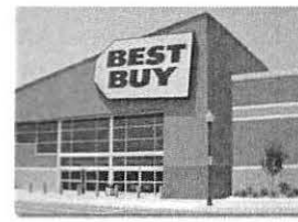
Right Generally Not Acceptable
