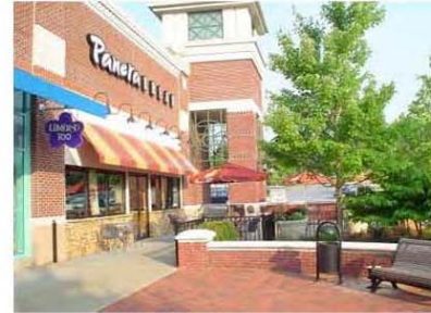
B – Example showing brick and precast
