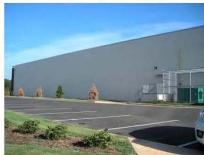
Figure 64 A – Not permissible
