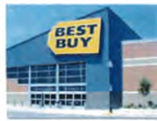
Right Generally Not Acceptable
