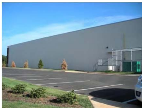
Figure 64 A – Not permissible
