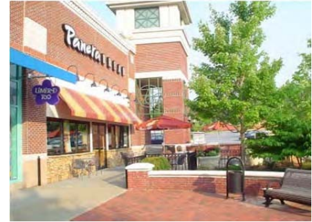
B – Example showing brick and precast
