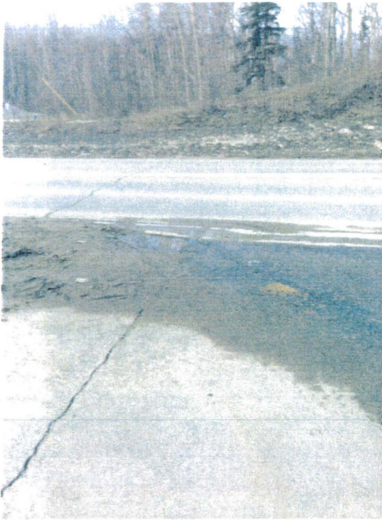
E Glen Cir Approach - South side
