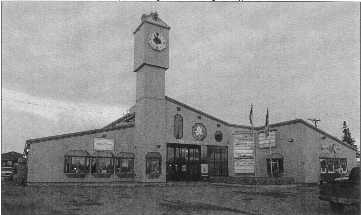
(front building elevations looking westerly)
