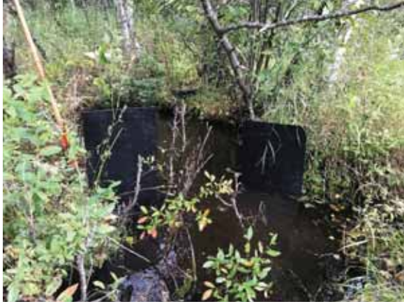
Photo 1: Installation of Weir 1
