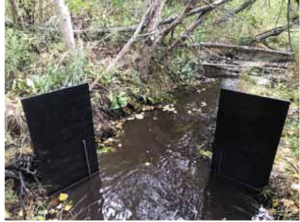
Photo 2: Installation of Weir 2
