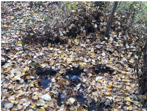
Photo 3: Sink hole covered with leaves
