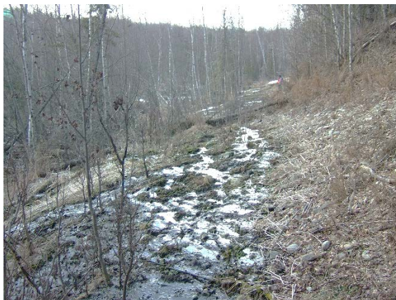
Leakage at Toe of Percolation Bed 3
