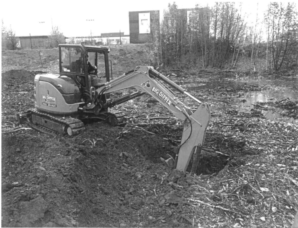
Excavator and ponding in NW of lot
