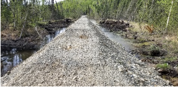
Photo 1: Looking South Down Berm
