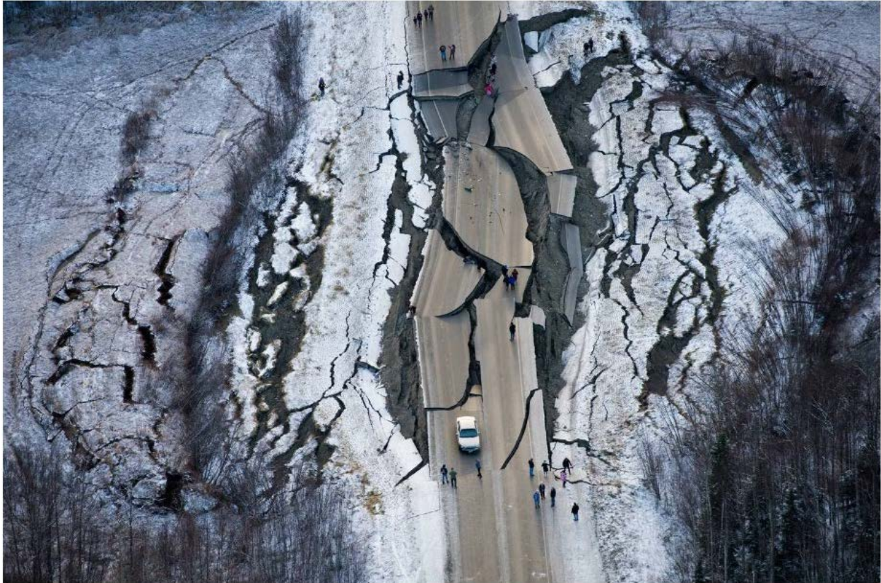
Figure 3-12 Lateral Spread of Vine Road, November 30, 2018
