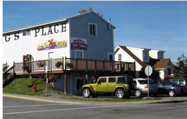
Land use patterns established by railroad surveyors in 1917 are highly visible today in the Downtown area.
