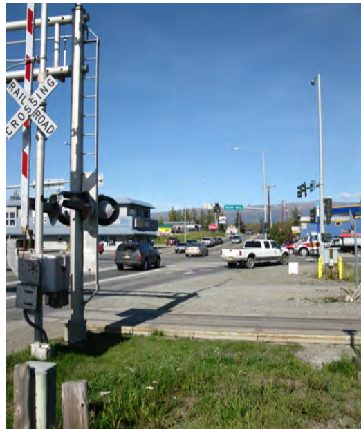
Rail crossing at Main and Knik Goose Bay Road.
