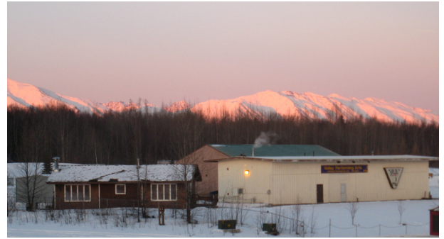
VPA owns its facility on land leased from the City of Wasilla. Its readapted buildings limit VPA's capacity to serve growing regional needs.
