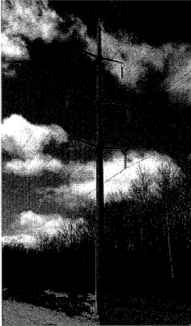
Typical double circuit 115/115 kV 115/115 kV steel davit arm structure
