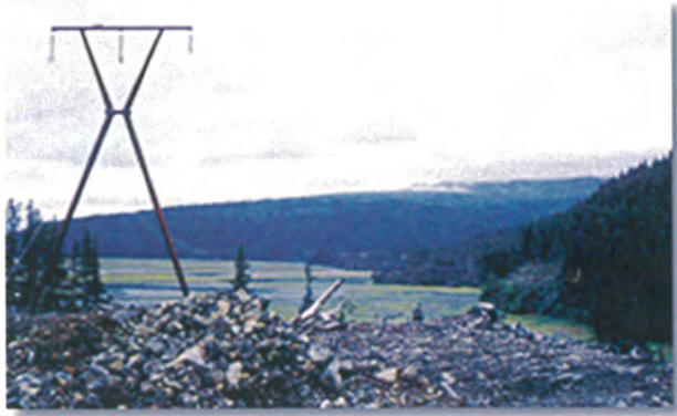
Bradley Lake Kachemak Bay 115 kV tubular X-tower (new construction)
