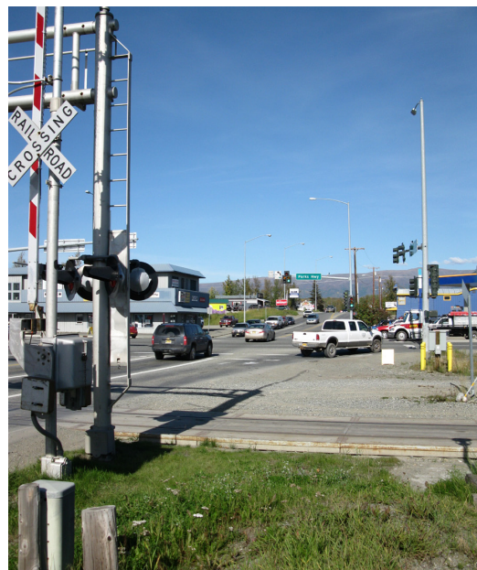
Rail crossing at Main and Knik Goose Bay Road.
