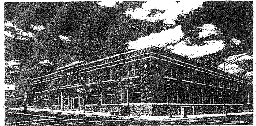
Figure 3-24. The Korger Building's development in 2004 involved the direct participation of seven different entities. Located in downtown Chippewa Falls, Wisconsin, it represents the combined efforts of a variety of local, state, and federal governmental organizations, in addition to the private sector. Source: Chippewa Falls Main Street, Inc.
